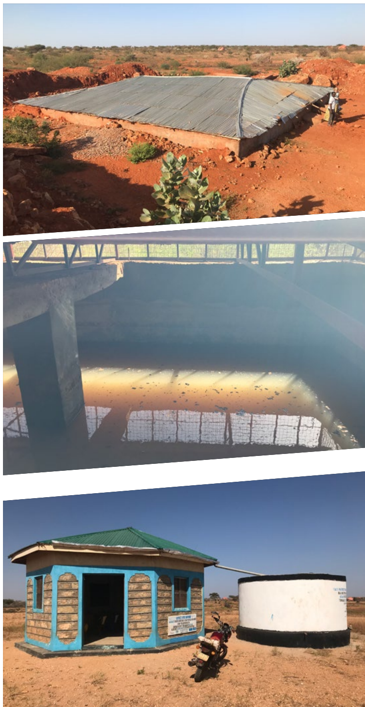
Figure 38. Rain Water Harvesting tank at the DRR centre of Daytuli community.
