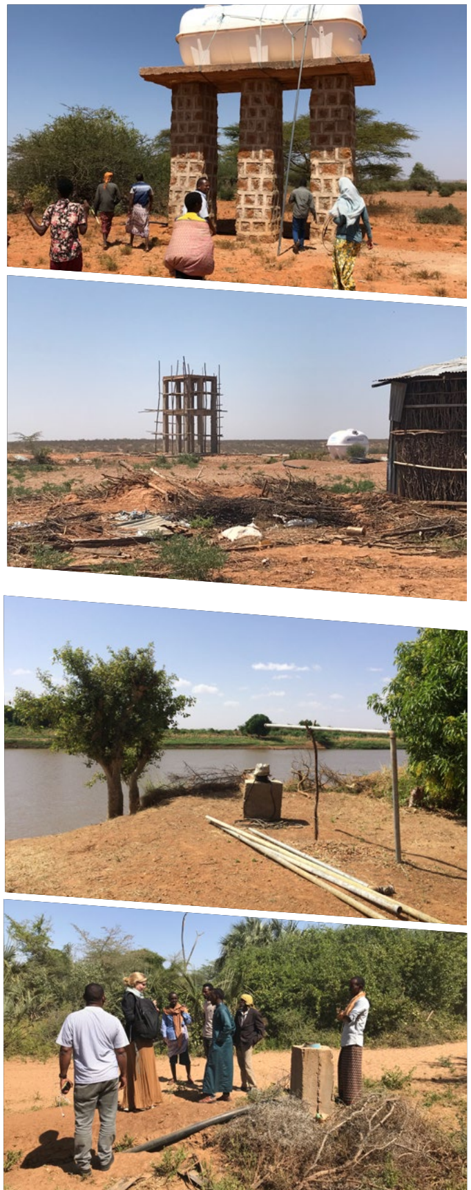
Figure 34. Third: The non-functional borehole at the Genale river bank, near Sigallow village. Below: the unfinished borehole near Holomoge village, at ~100 m from the Dawa river.
