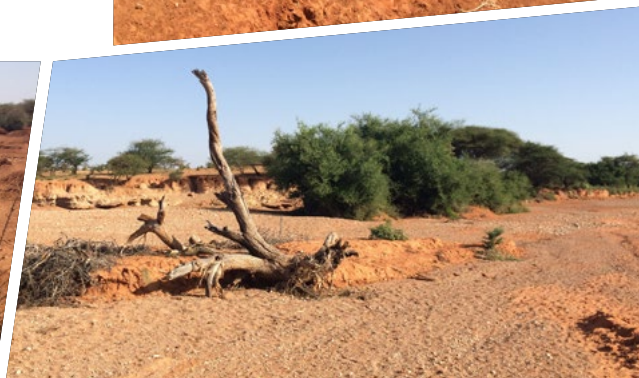
Figure 22. Above: Severe gully erosion in Biyoley kebele exposing hardrock beneath. Below: erosion of wadi banks in wadi with coarse sediment.
